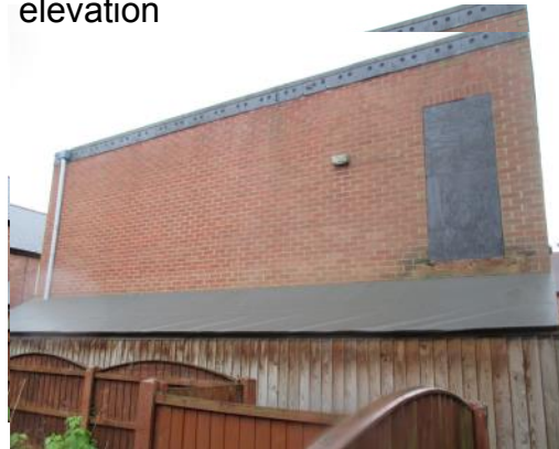
Image 4: Side (north west) elevation
